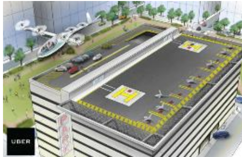
Figure 2.53 - Top of an eight-story downtown parking garage converted to vertiport capable of supporting 12 VTOLs.
