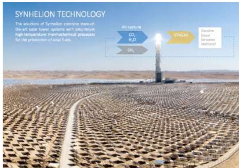
Figure 19.38. IMAGE@Synhelion – A solar field of mirrors and tower for solar jet fuel production would look like today's tower CSP projects
